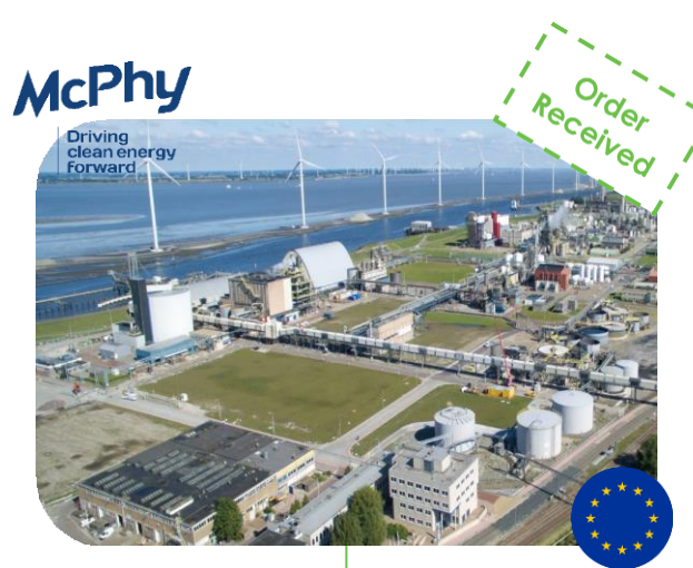
Delfzijl Industrial Park – The Netherlands
